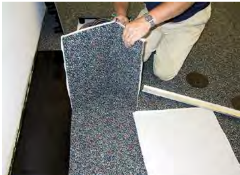
Cutting carpet tile for perimeter
