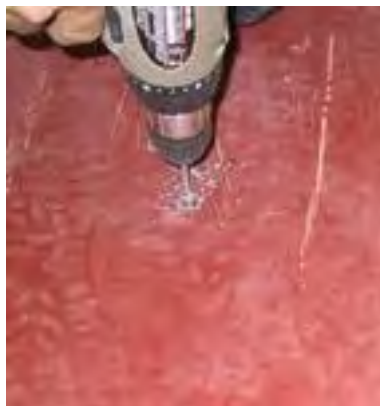
Drilling Ramp for countersunk anchors
