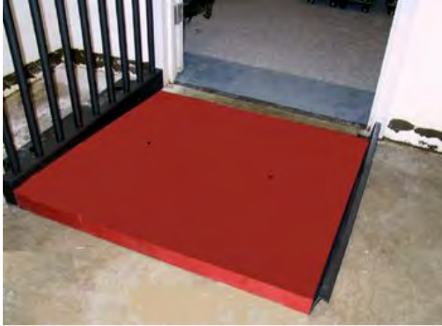
One Piece Ramp Installed with Rail and Z Trim
