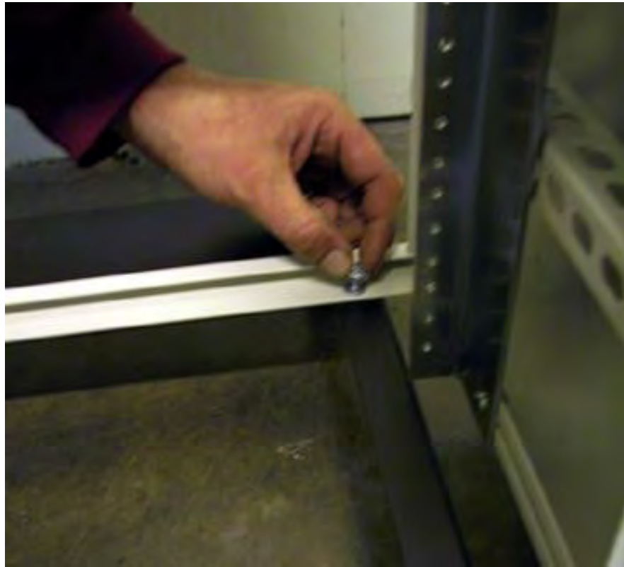
Picture 10-5 Installing LDS Cabinet to Base Unit
