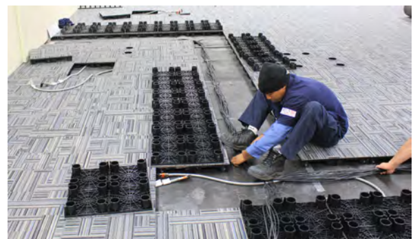
Picture 10-15 Opening Up Floor and placing Bundled Cables on Sub-Floor
