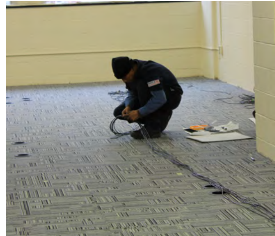
Picture 10-14 Rolling Out & Sorting Cabling on Top of Floor and Tie Wrapping as Required
