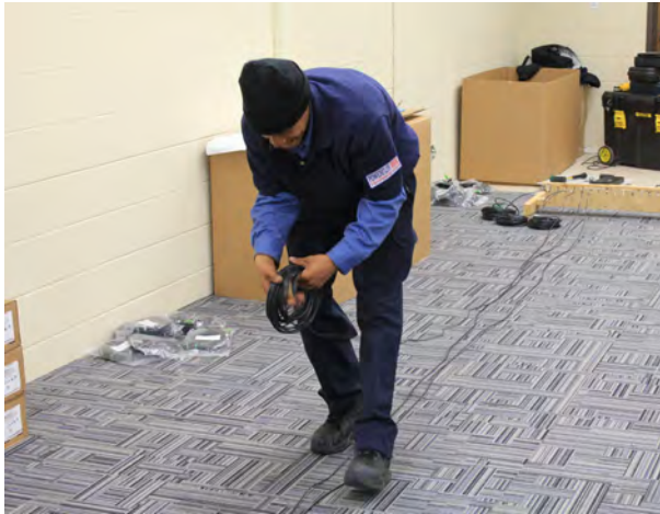
Picture 10-14 Rolling Out & Sorting Cabling on Top of Floor and Tie Wrapping as Required
