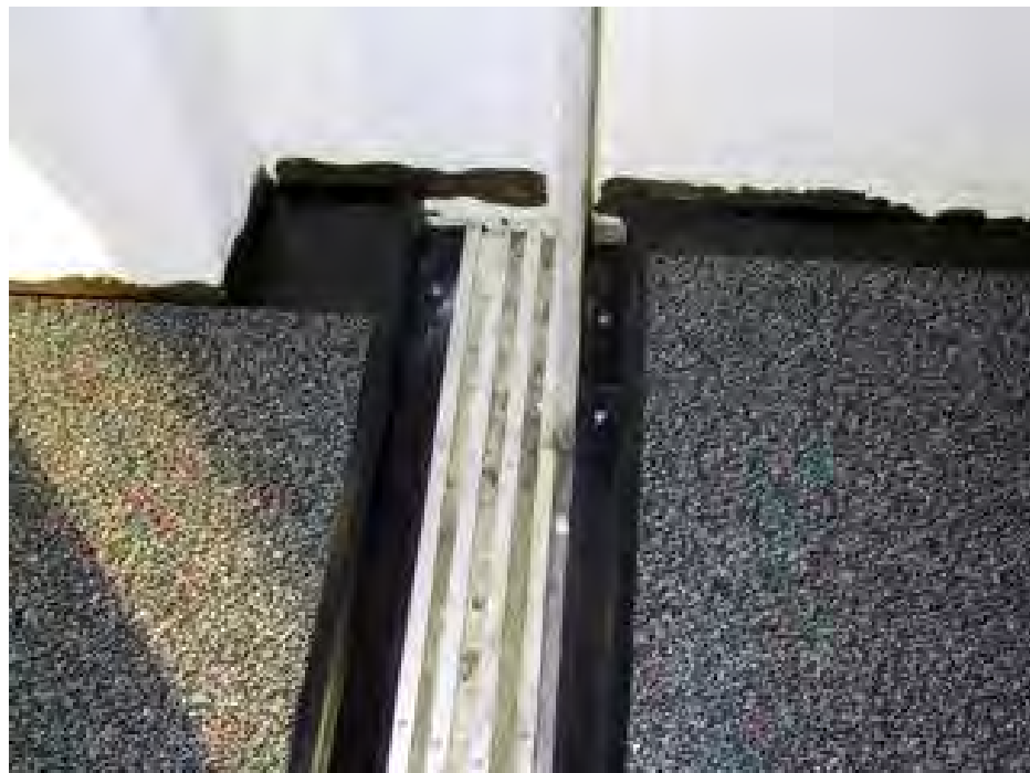
Picture 7-15 Z Trim Installed
