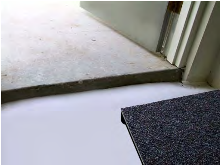
Recessed Sub-floor with full panels requiring perimeter filler
