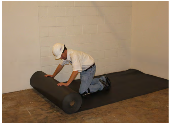
Picture 5-1 Foam Rolls / Installing Foam Underlay
