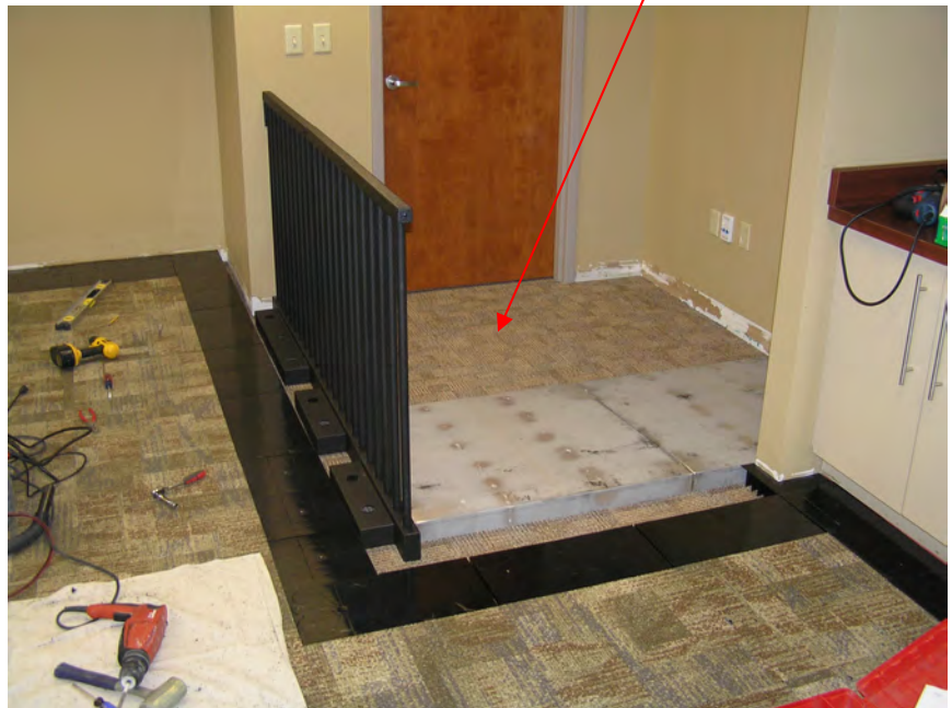
Drilling Ramp for countersunk anchors
