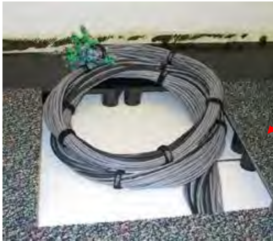
LDS with Data Cables fed through base
