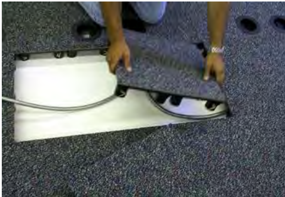
Picture 9-17 Installing completed panel into system
