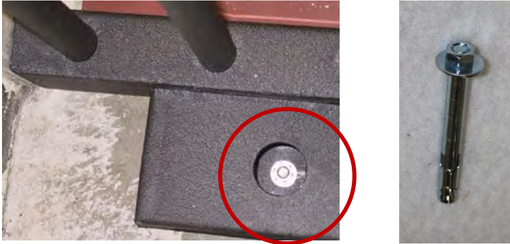
Picture 8-8 Rail anchored to floor with 3" x 3/8" anchor bolt
