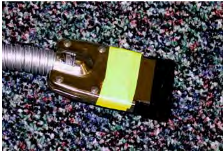
Picture 9-15 Completed Color Coding of Cable Assembly
