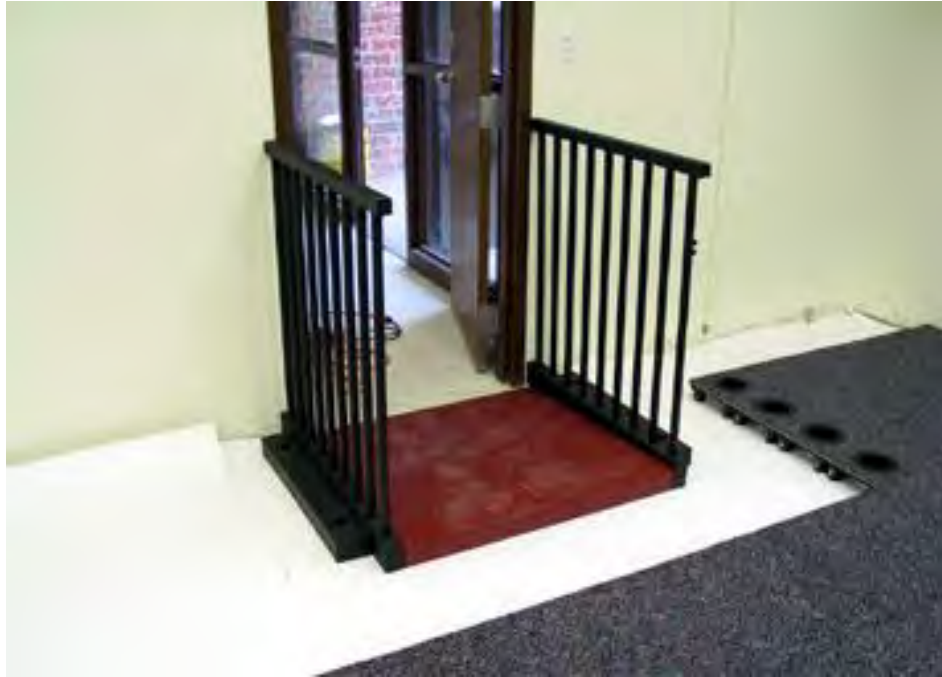
Rails located both sides of ramp
