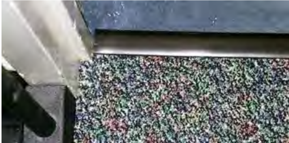
Installed Transition Molding
