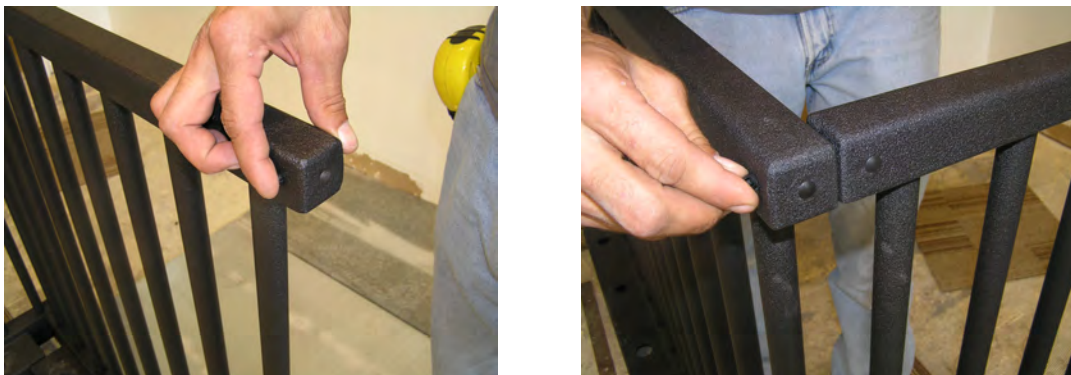
Picture 8-10 Rail Top Cap Holes are filled with Plugs
