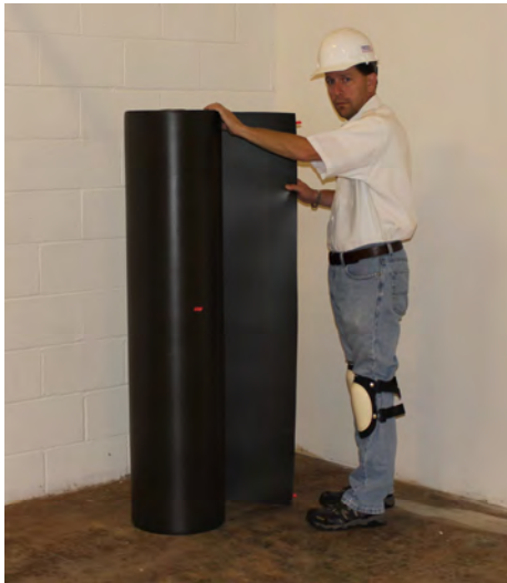
Picture 5-1 Foam Rolls / Installing Foam Underlay
