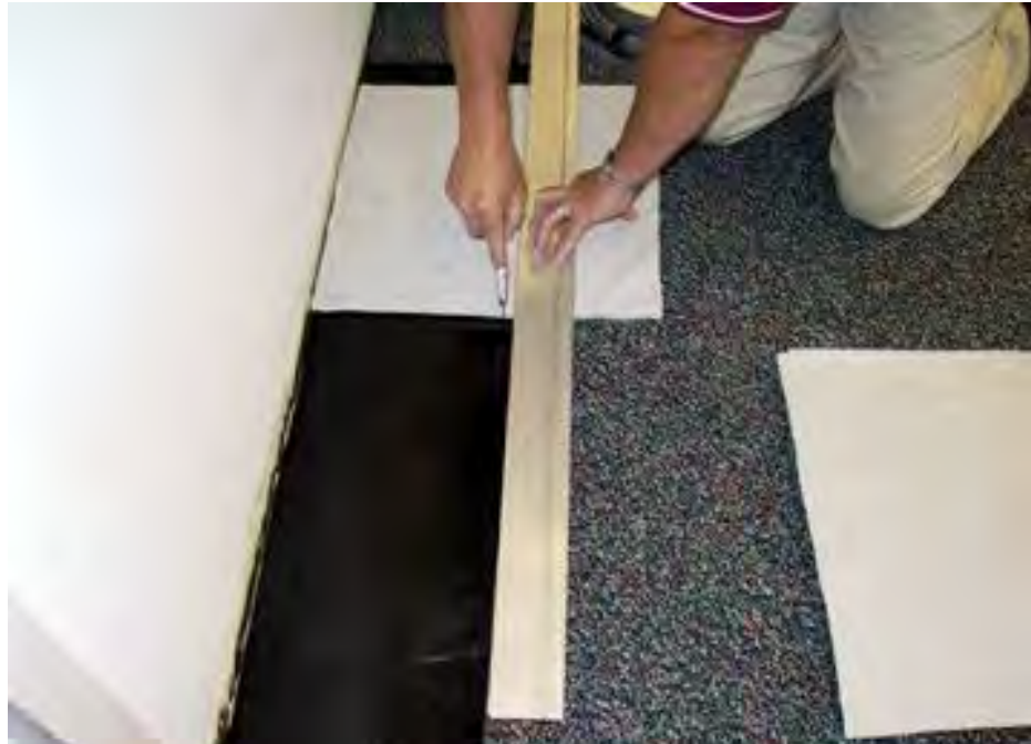
Cutting carpet tile for perimeter
