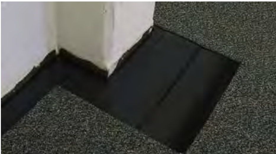
Picture 7-8 Filling in Perimeter around obstacles
