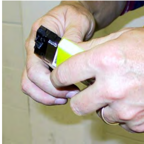
Picture 9-14 Applying Color Coding
