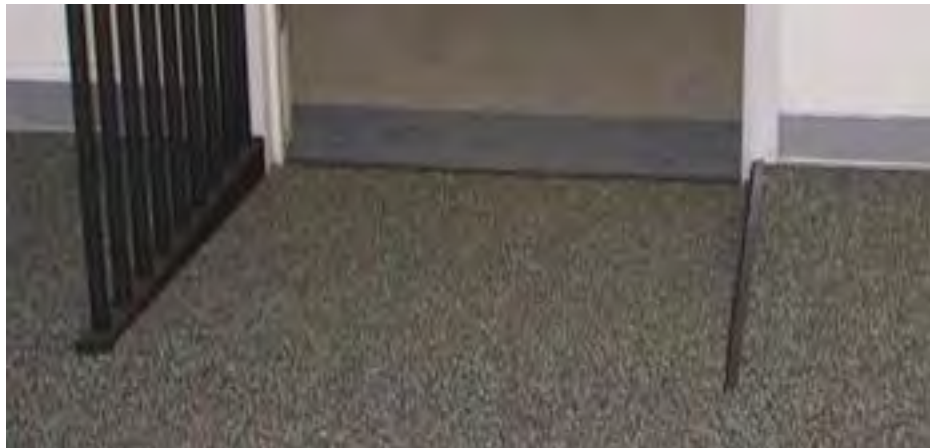
Completed Ramp / Rail Access
