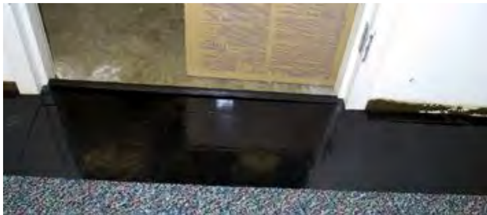
Z Trim / Perimeters in a doorway
