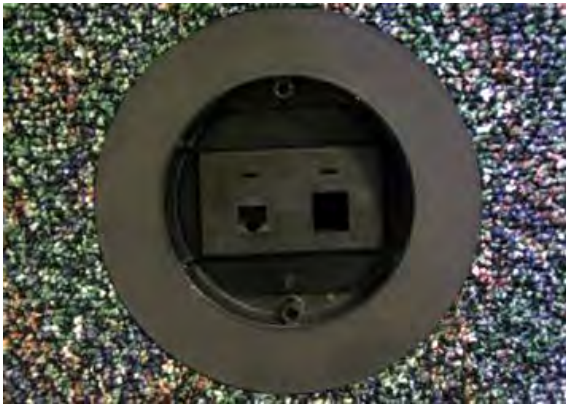
Completed Adaptor Plate Outlet
