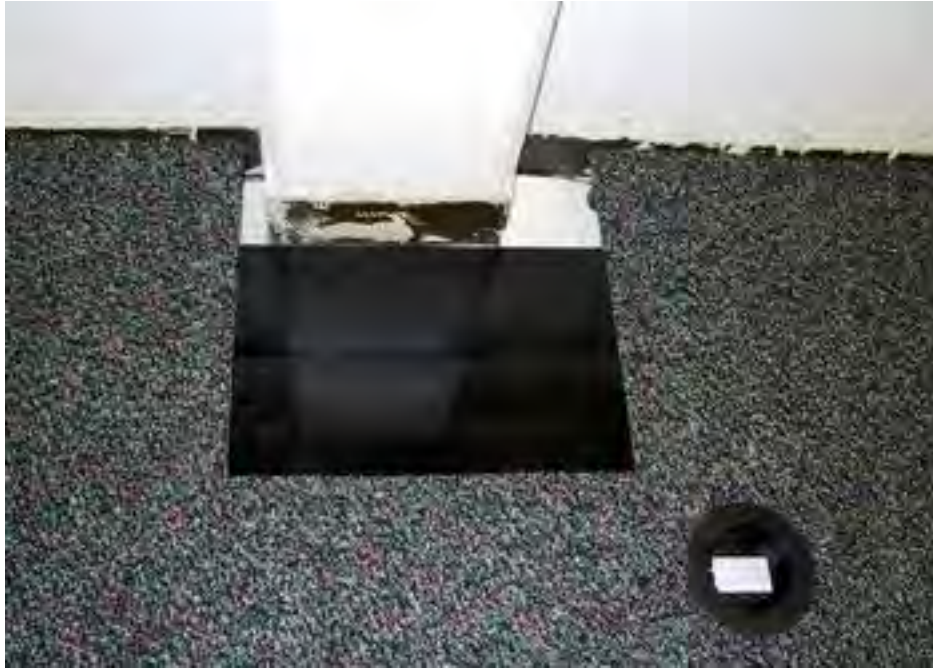
Picture 7-8 Filling in Perimeter around obstacles
